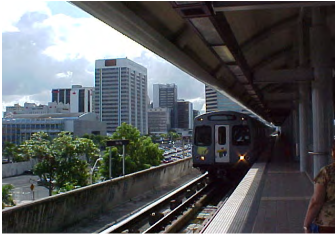
FIG. 10. TREN URBANO (SUBWAY), SAN JUAN. PHOTO BY AUTHOR. JANUARY 2006.
